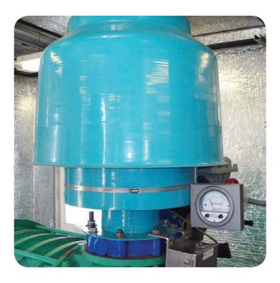
**Left:** Blower building interior with Endustra Tri-Vent® P09 intake filter silencer and differential pressure gauge at the Metropolitan Syracuse WWTP.
